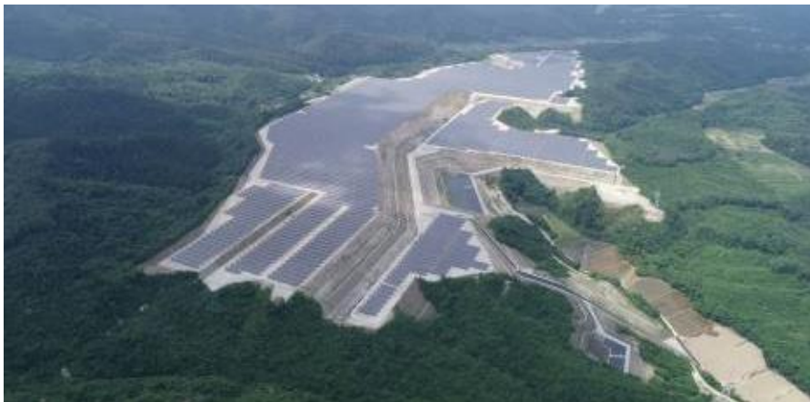
28MW solar power plant in Miyagi Prefecture
